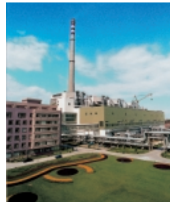
Beijing thermal power plant
